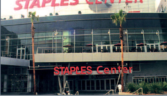
Installation by Giroux Glass, Los Angeles, CA.
