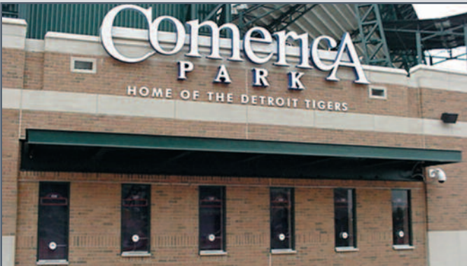
Installation by Universal Glass and Metal Inc., Detroit, MI.
